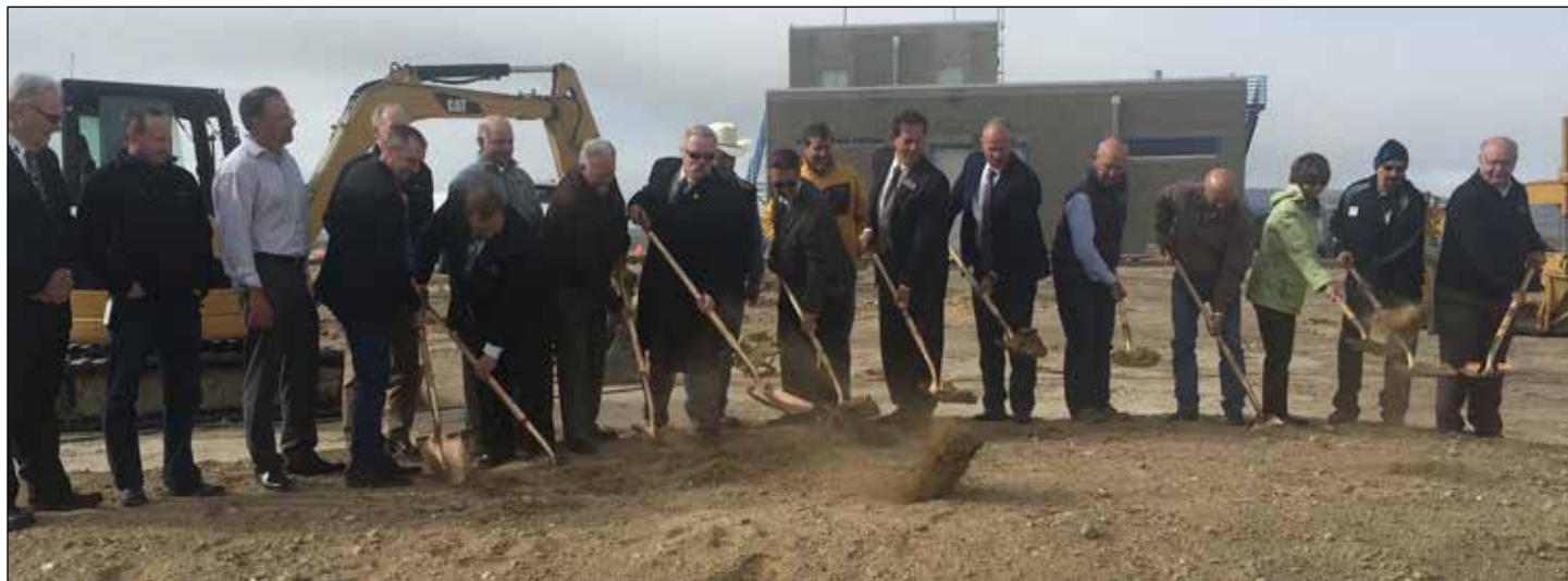
Wyoming Gov. Matt Mead helped break ground on the new terminal and hangar in Rock Springs on June 13.
