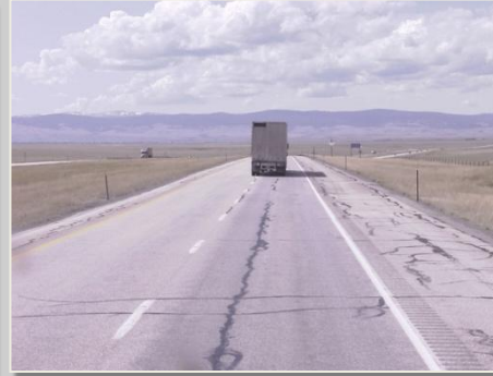
Cracking
