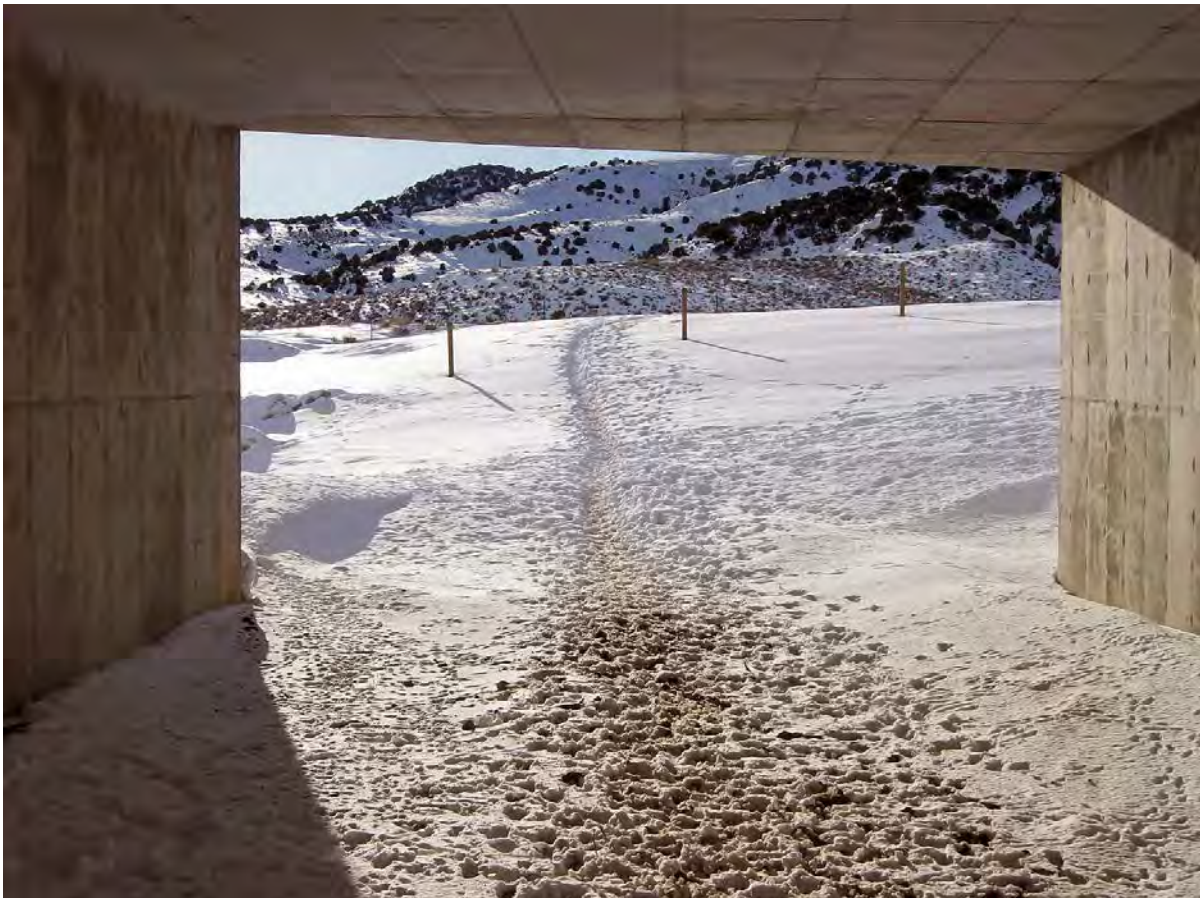
Figure 2. View, facing west, of the deer trail through the underpass.
