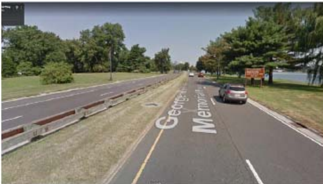
George Washington Parkway, 11' travel lanes, 1-2' shoulders, 13' grassy median, 40 MPH speed limit
