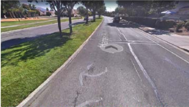
Harden Parkway, Salinas, California, 12' left travel lane, 11' right travel lane 4' right shoulder, No left shoulder, 18' grass median, 35 MPH speed limit
