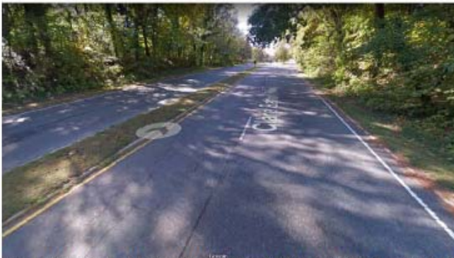
Clara Barden Parkway Maryland, 11' travel lanes, 6" left shoulder, 2' right shoulder, 10 median, 45 MPH speed limit
