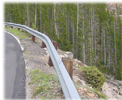
Existing guardrail does not meet safety standards.
