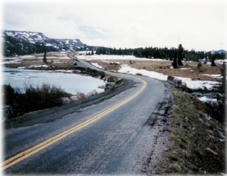
Narrow travel lanes contribute to pavement edge breakup from wider vehicles.
