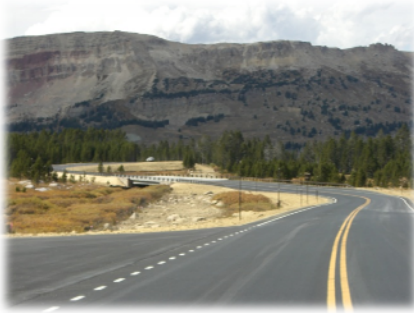
Completed Section of Segment 4 Little Bear Creek Bridge 1 Top of the World Store Beartooth Highway
