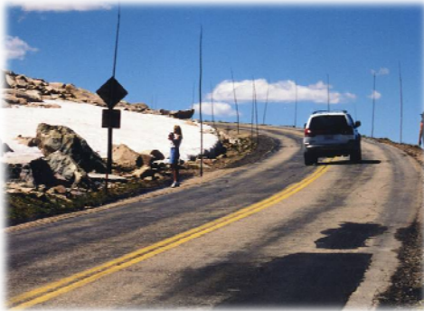
Narrow travel lanes with no shoulders pose a safety hazard to motorists and pedestrians. Poor drainage causes lack of surface support and deterioration.
