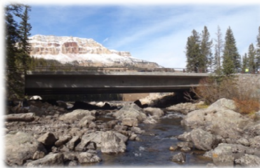
FY 2009 TIGER Completed Section of Segment 4 Beartooth Lake Outlet Bridge Beartooth Highway
