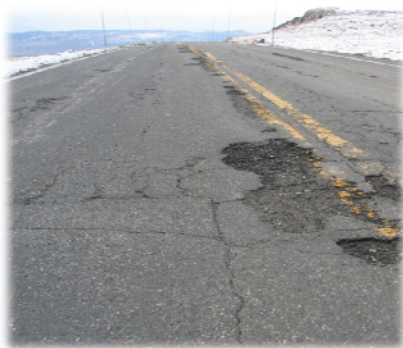
The current pavement condition index of 40 requires major reconstruction.
