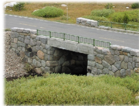
Existing bridges are in disrepair and rated functionally obsolete.
