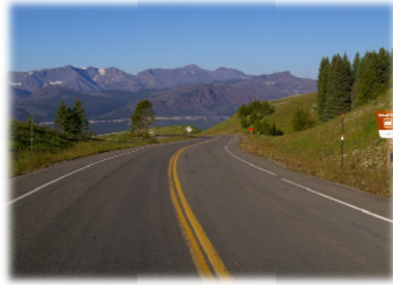
Completed Section Typical of Segments 2 and 3 Beartooth Highway
