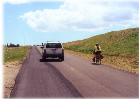
Existing road width does not safely accommodate bicyclists.
