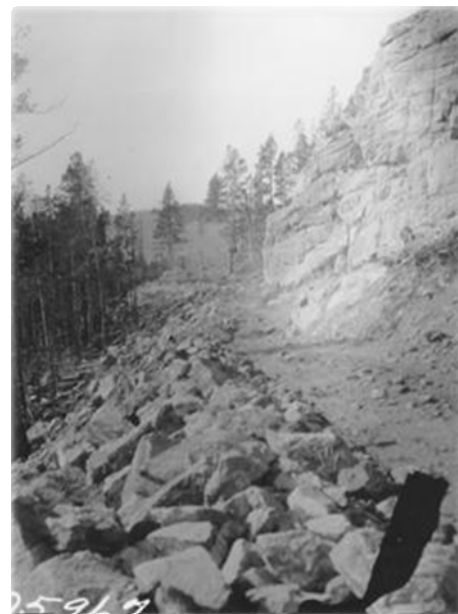
Beartooth Highway Construction, 1931
