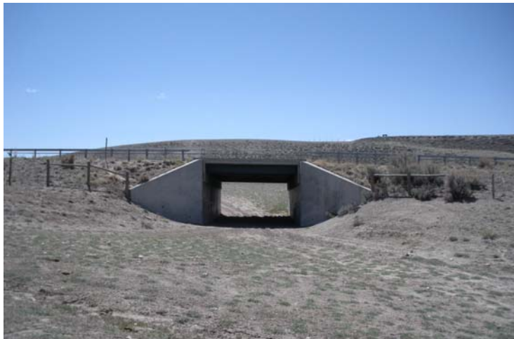
This structure is an example of a simple span bridge underpass facility.
