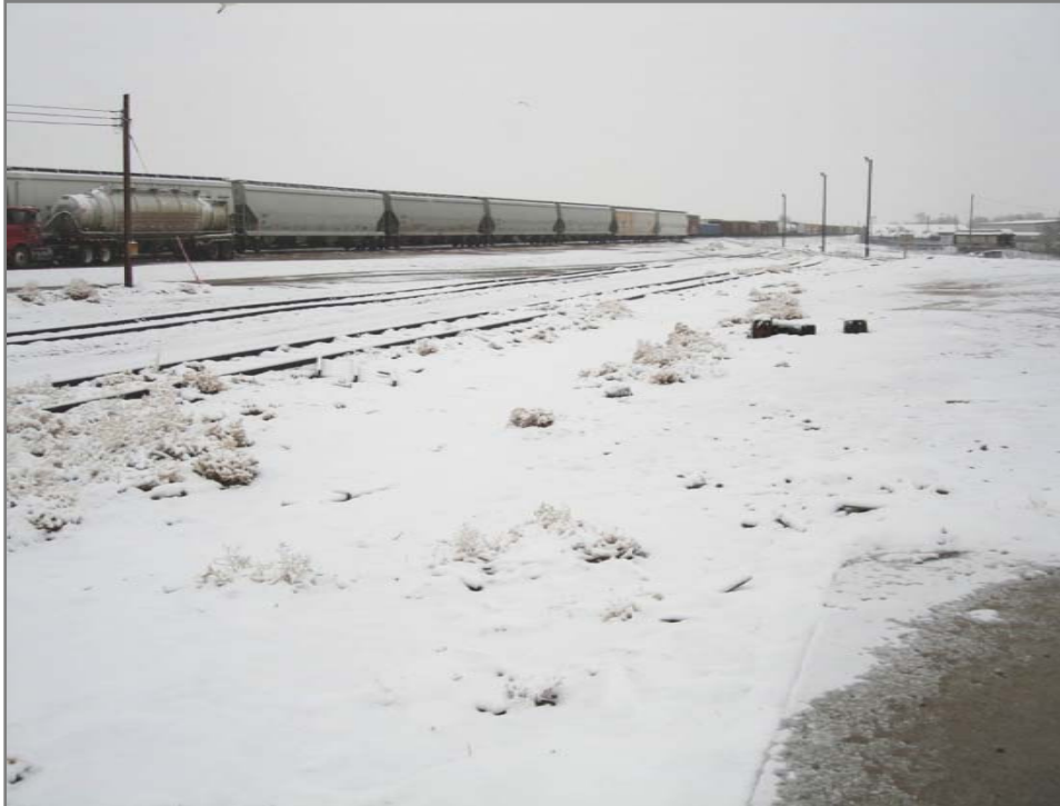
Detail view of east end of Casper Station for potential passenger train storage and platform site. Turn-a-round services could be performed to passenger train equipment in this area.
