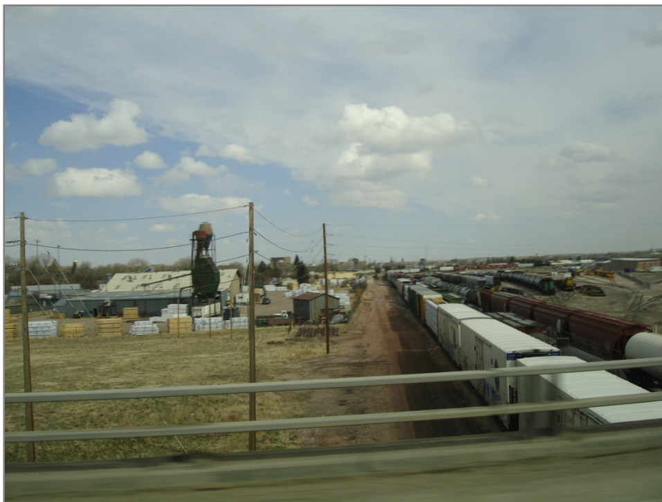
BNSF Cheyenne Yard. Freight congestion issues are shown. May be necessary to construct by-pass track for passenger train use for service to Casper.
