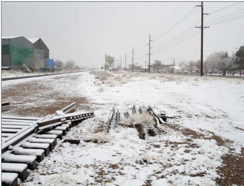
Evansville at Curtis Street – Looking West at potential suburban station stop for Casper.
