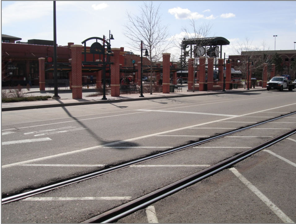
Fort Collins Intermodal Transportation Center BNSF Track in the middle of Mason Street
