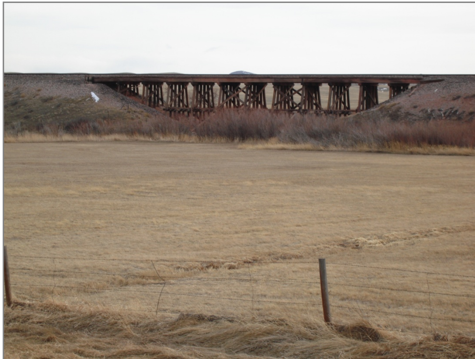
Wood Piling Trestle over South Fork of Horse Creek.
