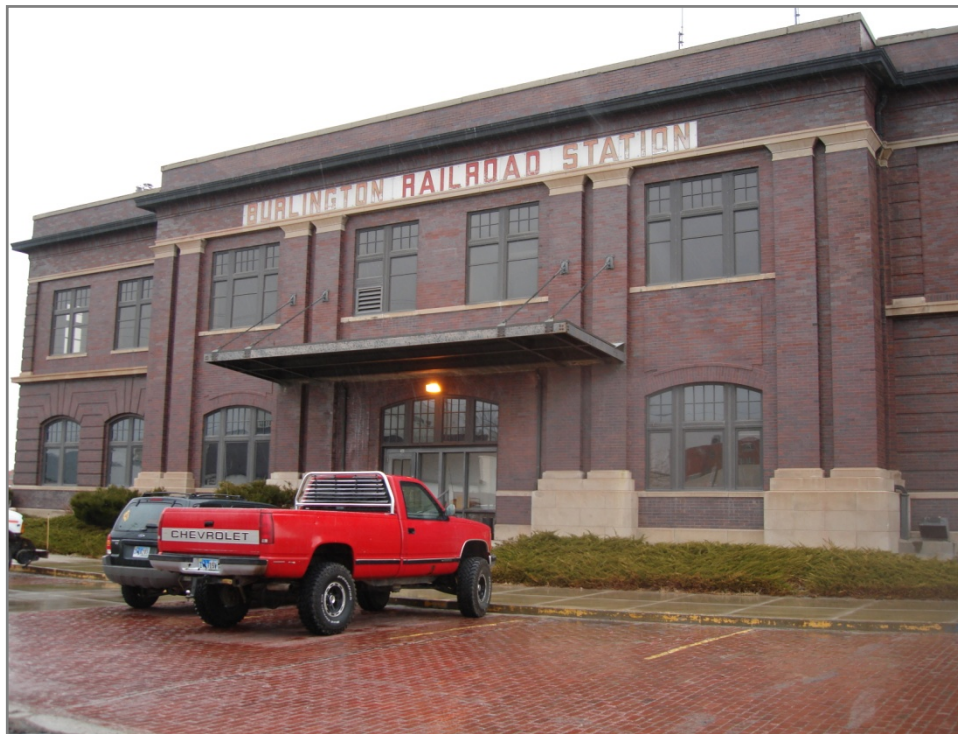
BNSF Administration Building at Casper. This structure was formerly utilized as station for Casper. Downtown District is one block south.
