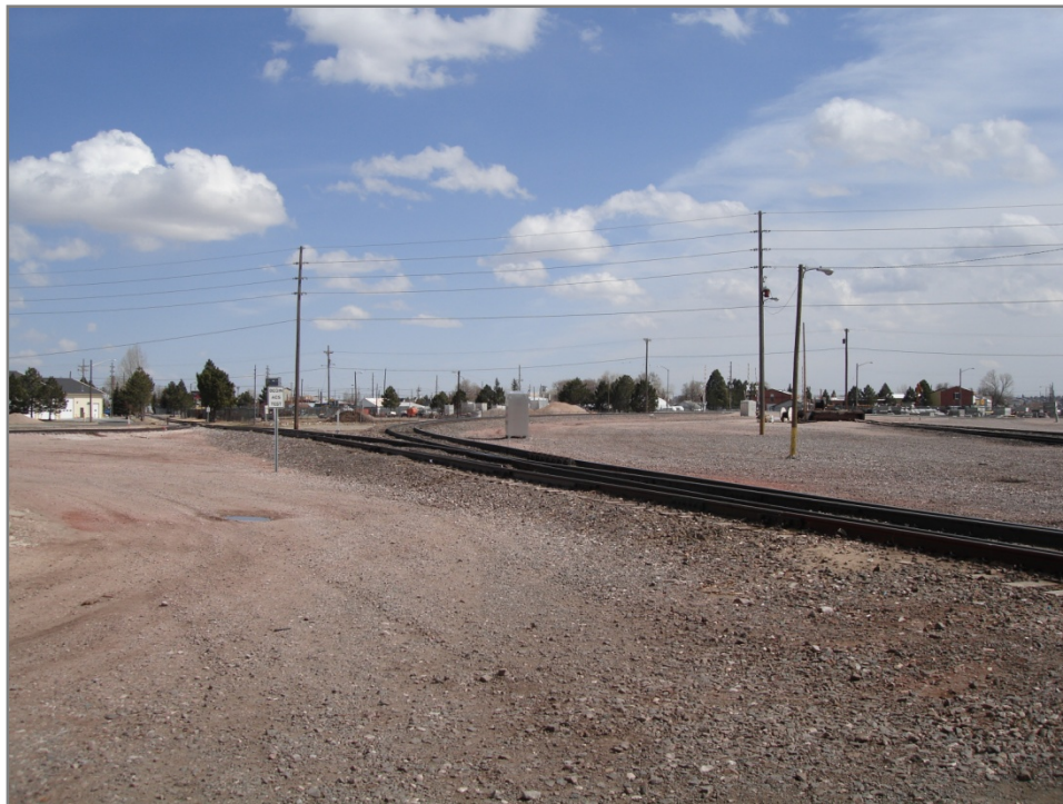
South End of BNSF Cheyenne Freight Yard. Potential passenger train storage location in center of picture.
