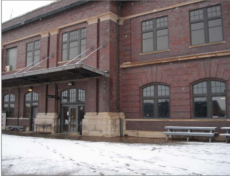
Station Track Side at Casper. Station Platform area in foreground.
