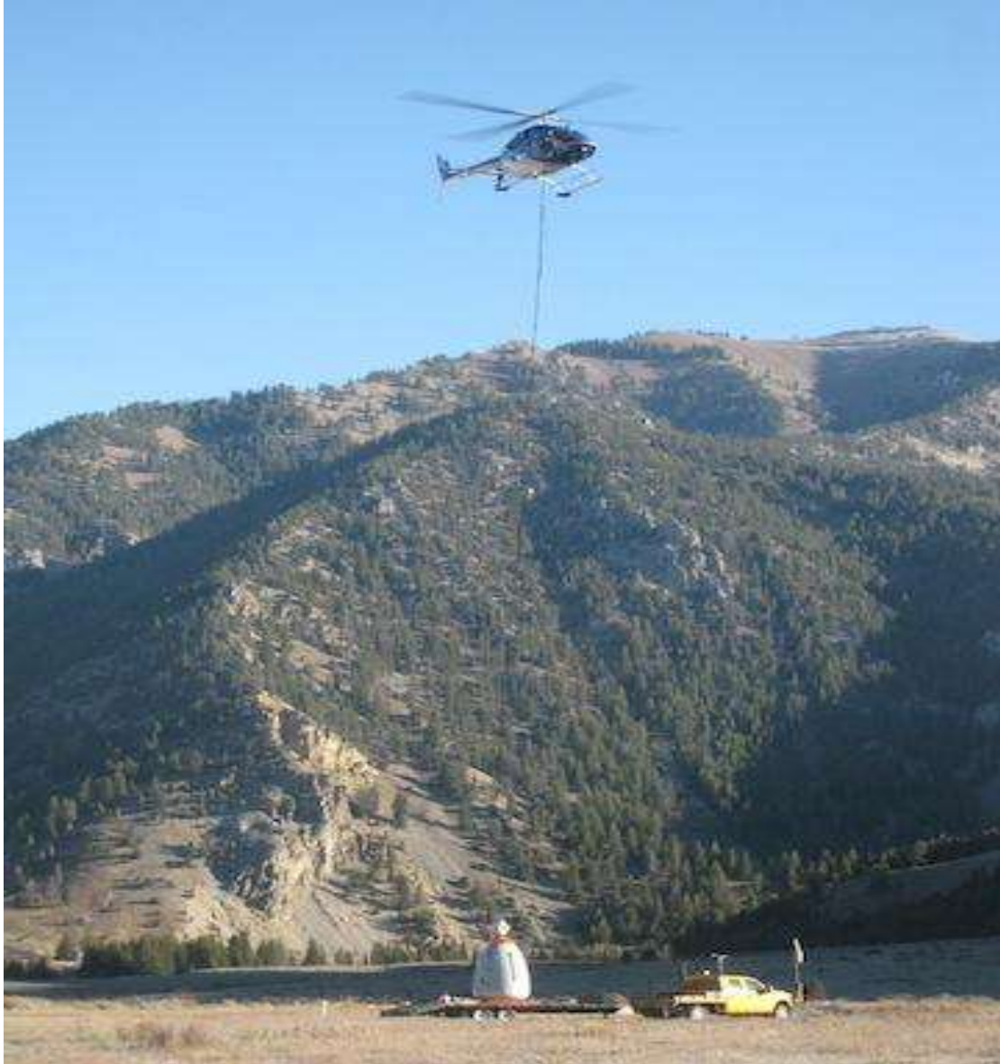
Figure 17. This is WYDOT’s first TAS O’Bellx® being lifted from the staging area for deployment in Hoback Canyon, Wyoming, above US Route 189/191.
