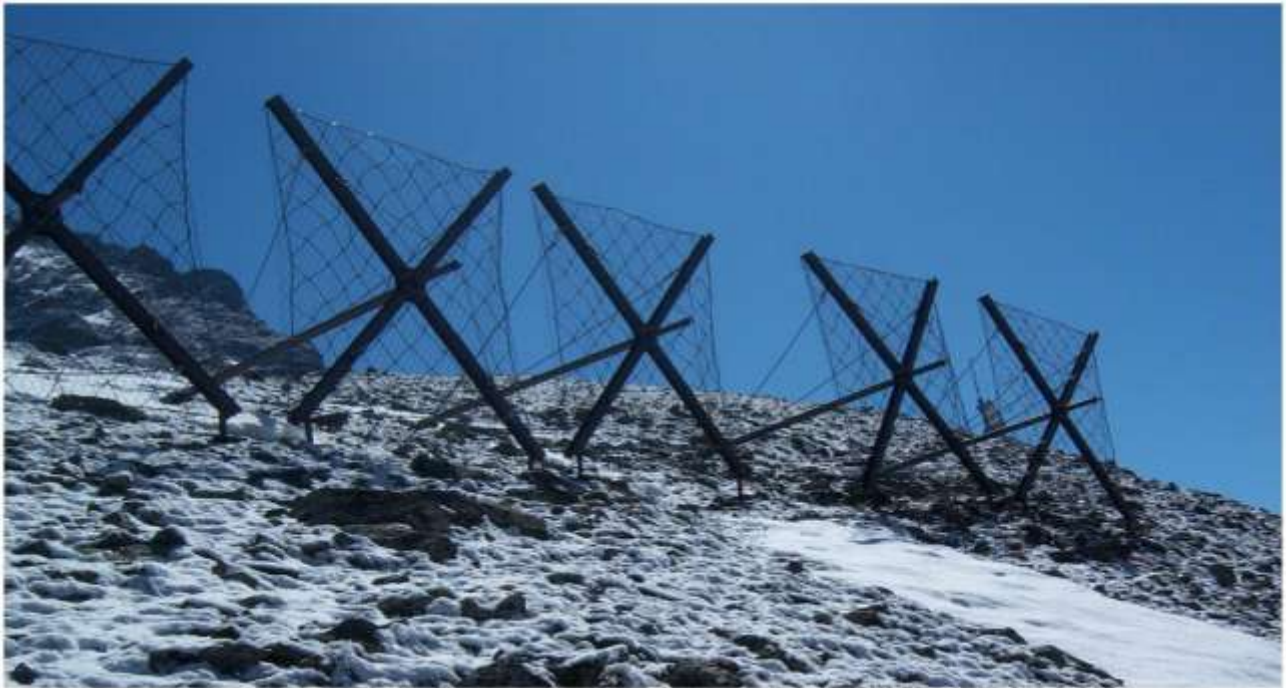
Figure 24. Snow-net snow supporting structures.
