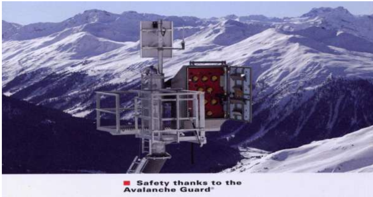
Figure 8. A Doppelmayr® Avalanche Guard® in the Austrian Alps in firing mode with its door open.
