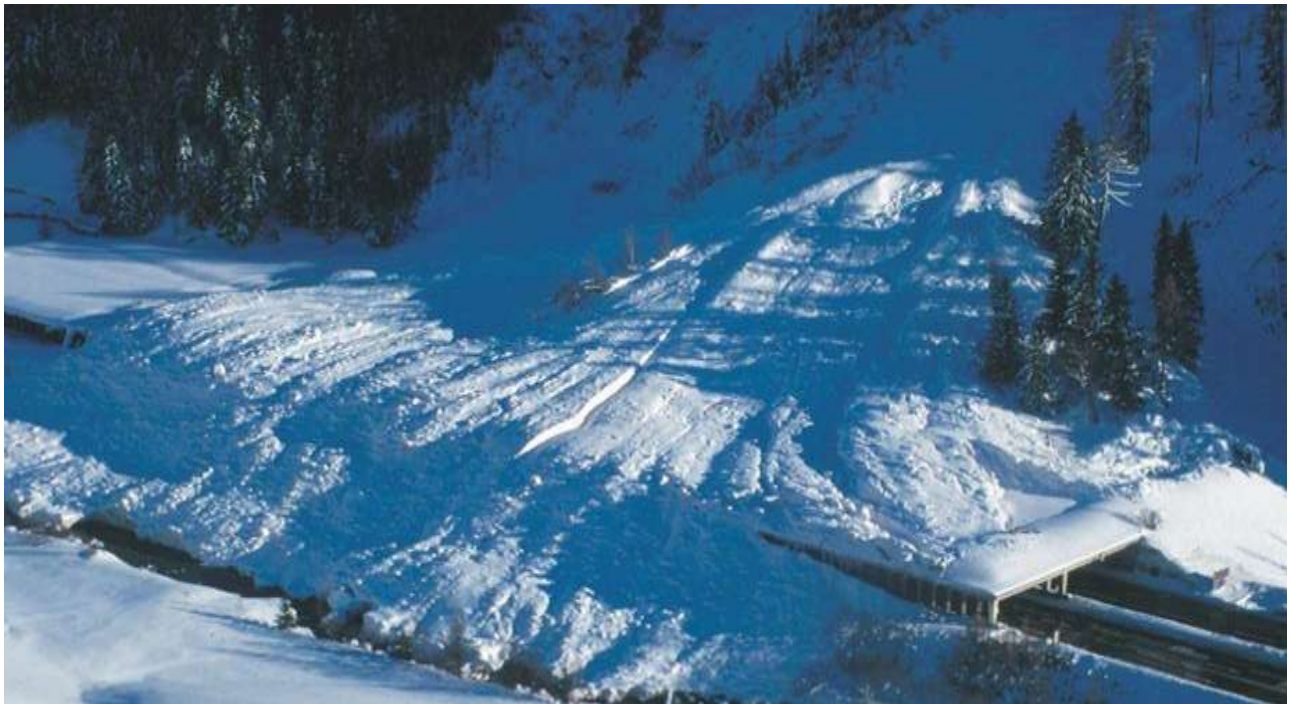
Figure 27. An avalanche shed defending a multi-lane, divided highway in the Alps.
