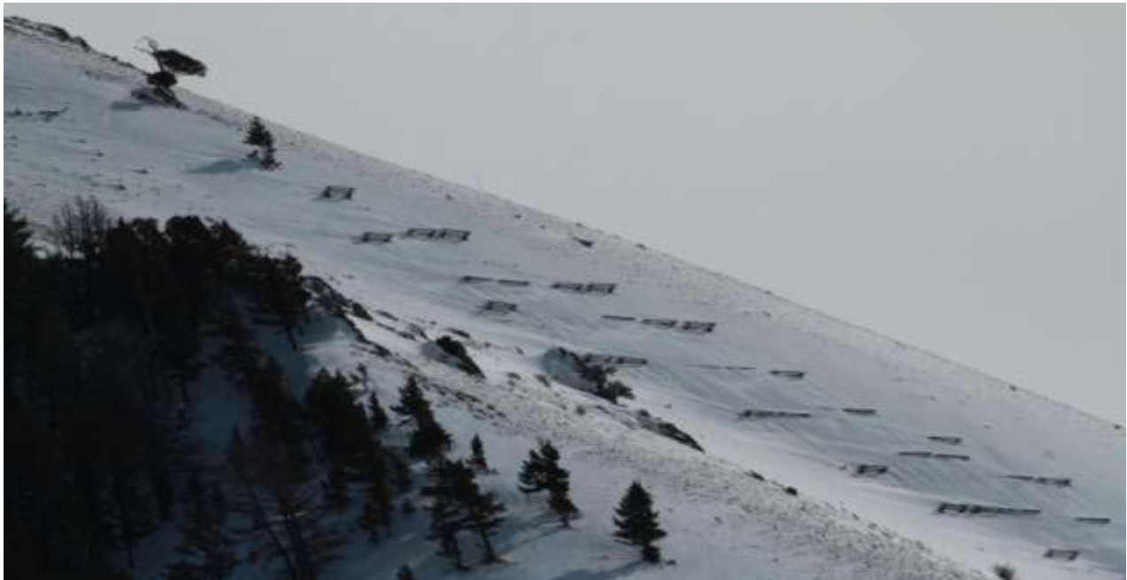
Figure 21. A snow supporting structure (a snow bridge, with horizontal members) being installed with a helicopter in the RM 151 Avalanche starting zone, above US Route 189/191, above the South Park area of urbanized south Jackson, Wyoming.
