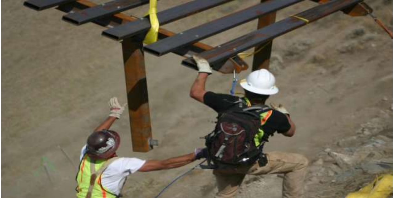
Figure 21. A snow supporting structure (a snow bridge, with horizontal members) being installed with a helicopter in the RM 151 Avalanche starting zone, above US Route 189/191, above the South Park area of urbanized south Jackson, Wyoming.
