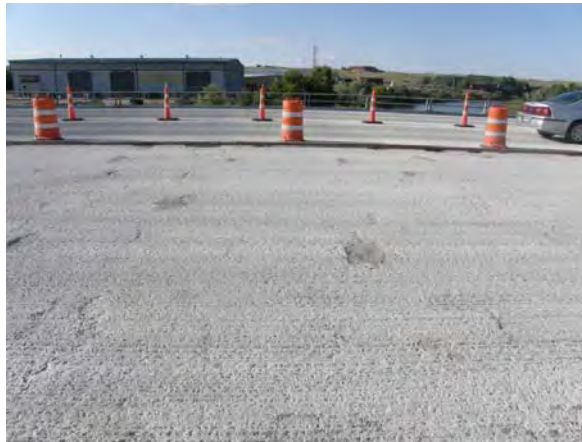
Figure 35: Casper Bridge milled surface (140 ft to 160 ft).
