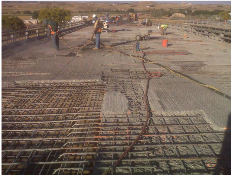
Figure 44: Douglas Bridge chipping looking east.
