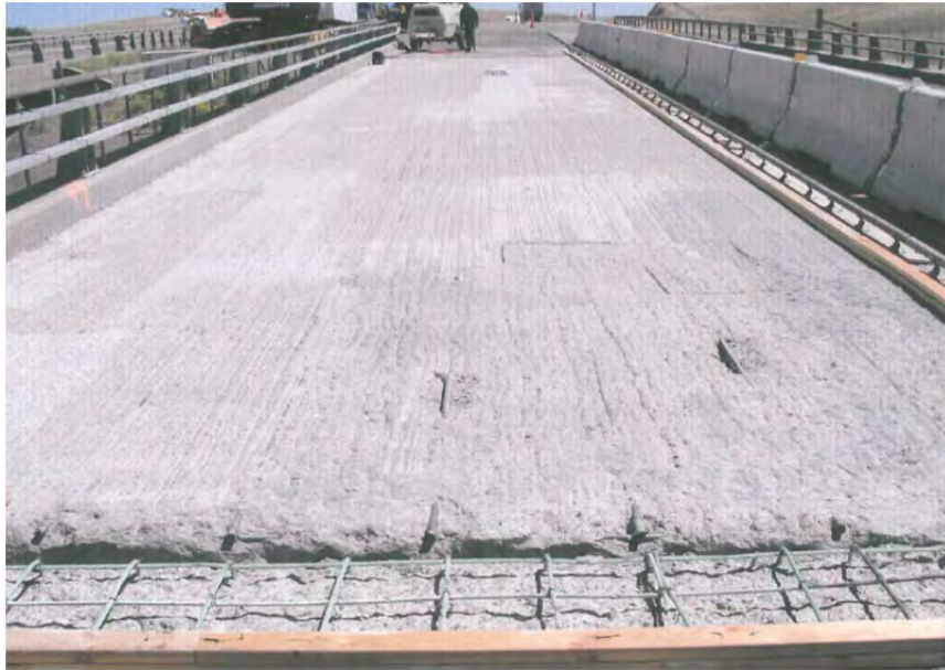
Figure 54: Remount Bridge reconstruction.
