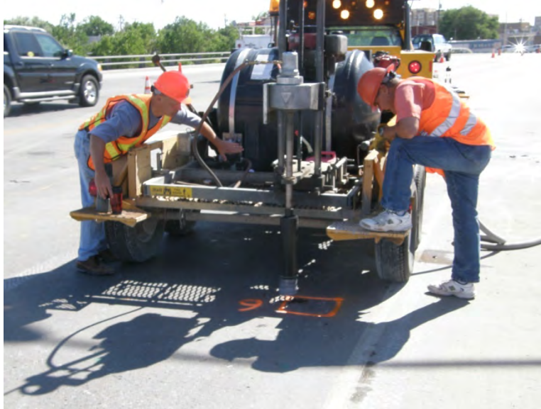
Figure 28: Coring rig on Casper Bridge.
