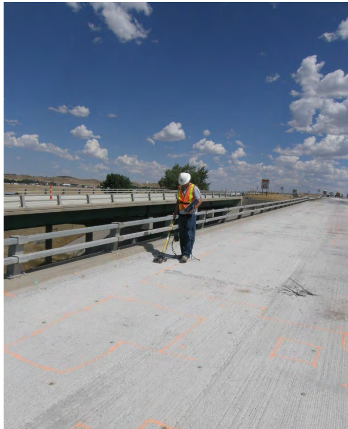
Figure 3 - GPR testing along the stripped surface of the bridge in Douglas Wyoming.
