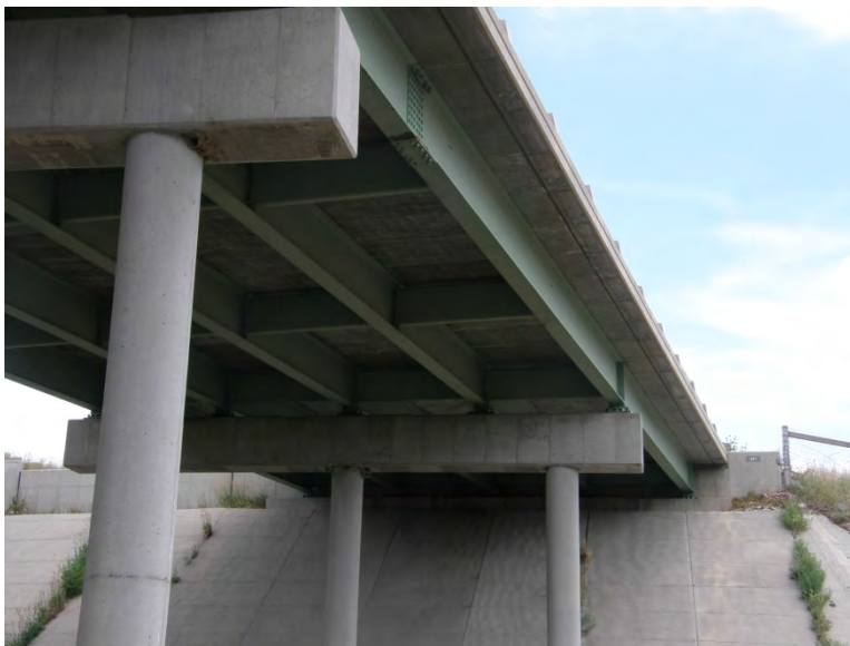
Figure 14: Southbound I-25 (Structure AFY) Bridge underside in Douglas, Wyoming.
