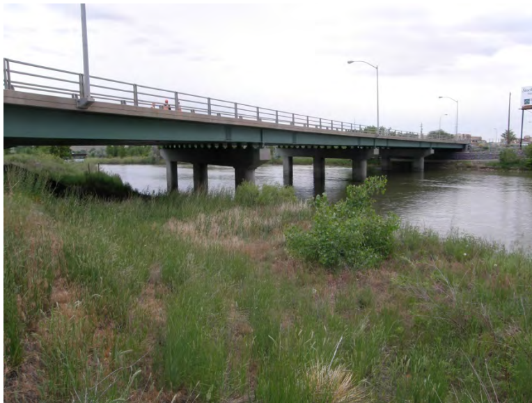
Figure 11: First Street Bridge in Casper, Wyoming.
