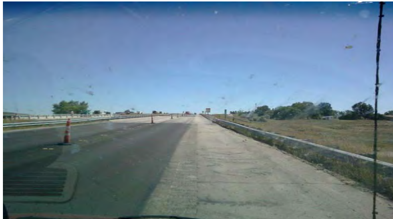
Photograph 1. Bridge on I-25 in Douglas, Converse County,
