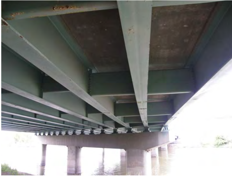
Figure 12: First Street Bridge underside in Casper, Wyoming.
