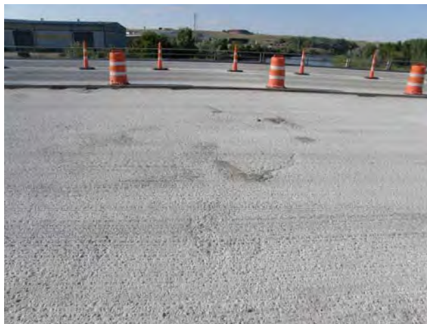
Figure 36: Casper Bridge milled surface (160 ft to 180 ft).
