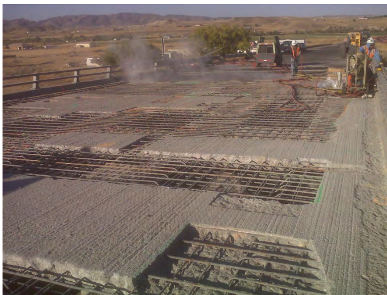
Figure 45: Douglas Bridge chipping looking east.
