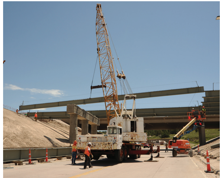
Bridge girders being placed in Pine Bluffs.
