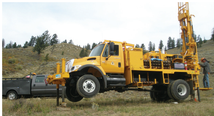
The Geology Program drilling at an on-site investigation.
