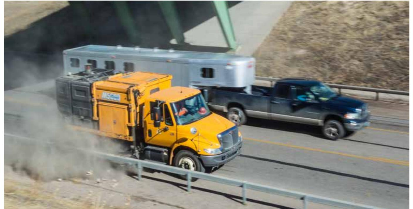
Wyoming Department of Transportation crews clean the shoulder below a bridge east of Cheyenne on Feb. 16. The crews clear the shoulder to increase safety and decrease potential for damage to the pavement created by moisture buildup.
