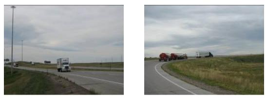
*I-80 is an important freight route.* On average trucks represent 50% of vehicles traveling through the *I-25/I-80 interchange.* The geometry of the loop ramps, short acceleration and deceleration lengths, and weaving conflicts make maneuvering large trucks particularly challenging.
