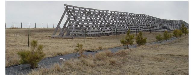
The use of a temporary structural fence with living snow fence promotes rapid tree growth and leads to earlier fence efficiency.
