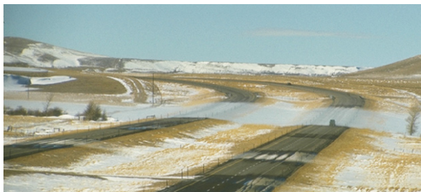
Structural snow fence is one of our most effective tools in fighting blowing snow
