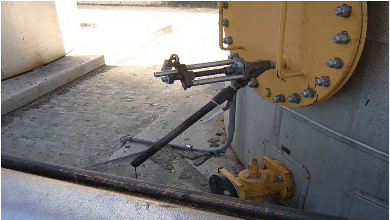
Figure 1 - Typical Sampling Valve for Tanker
