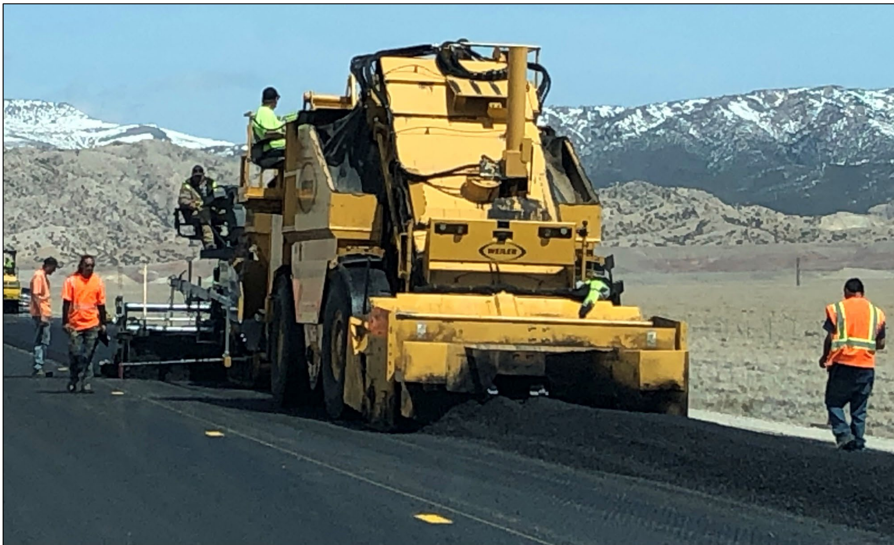
US20/WY789 pavement overlay work, north of Shoshoni, 4/2022
