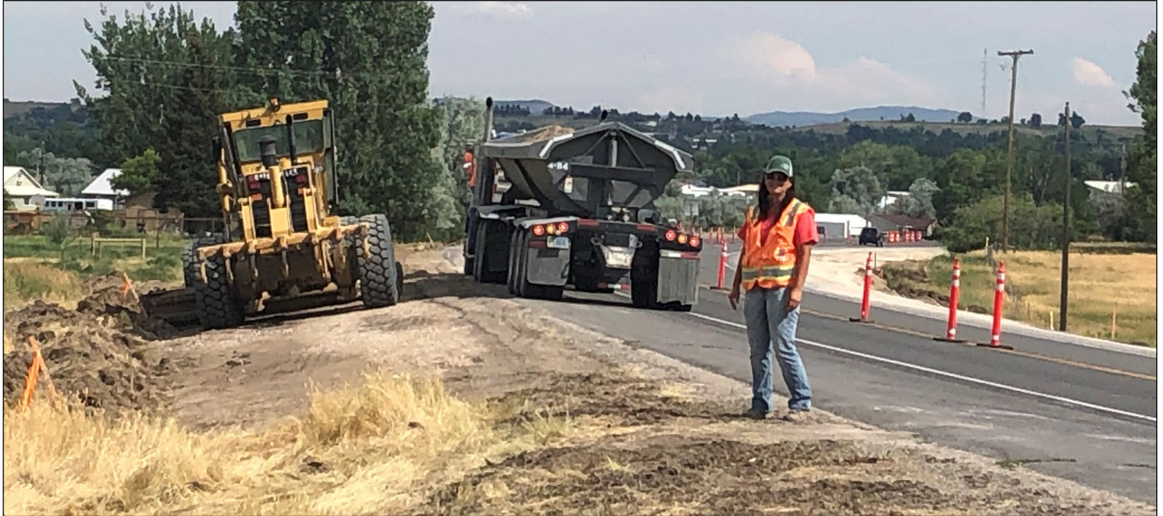
Slope flattening, north of Lander, 7/2022
