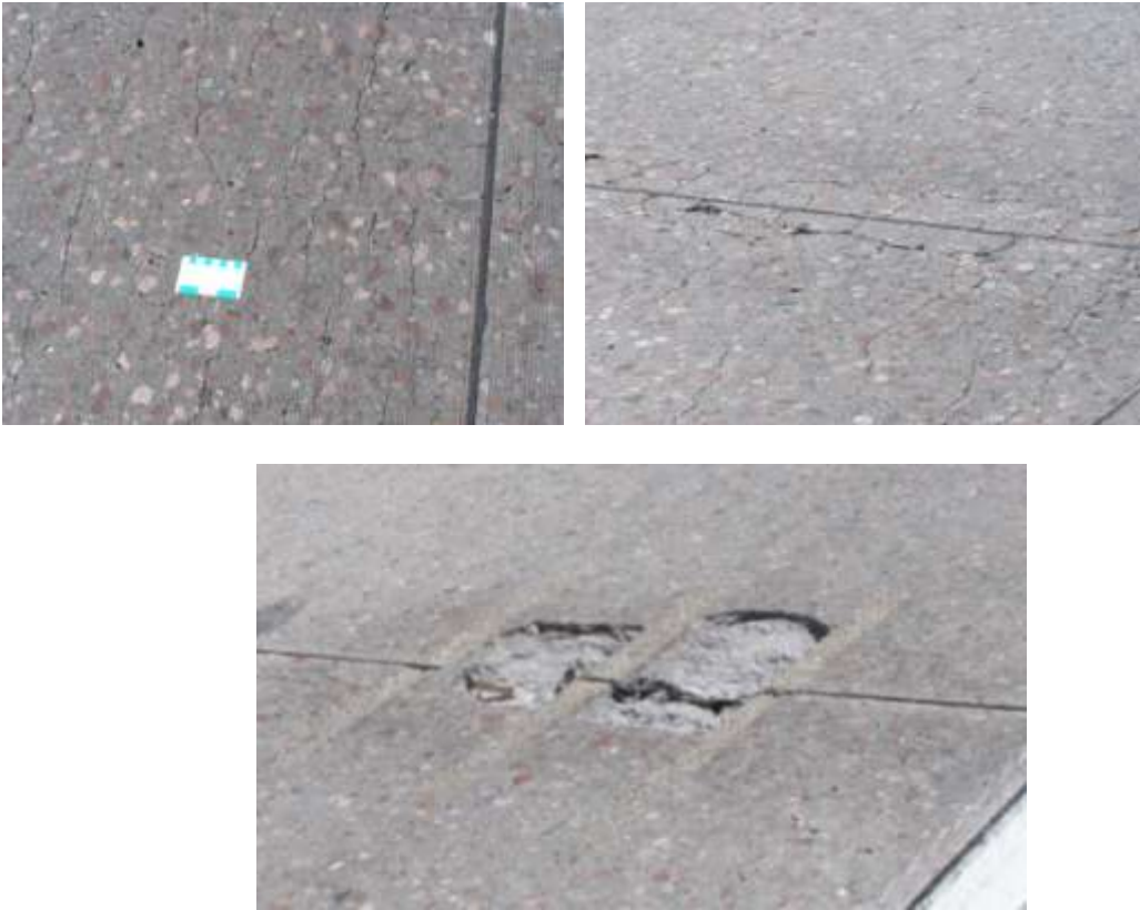
Figure 3. ASR damage on Interstate 80, east of Cheyenne a) general ASR map cracking, b) pop-outs combined with map cracking, and c) concrete failure between dowel bar retrofits is attributed to ASR.
