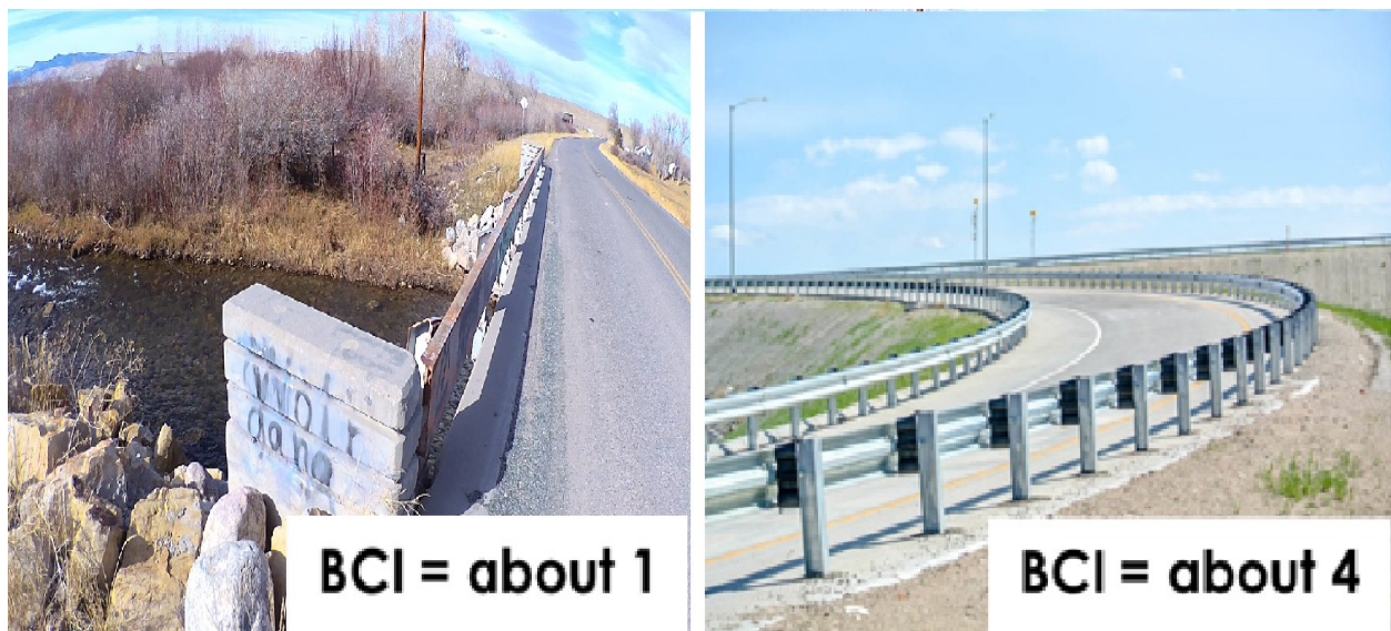
Figure 5. An example of the proposed BCI rating system.
