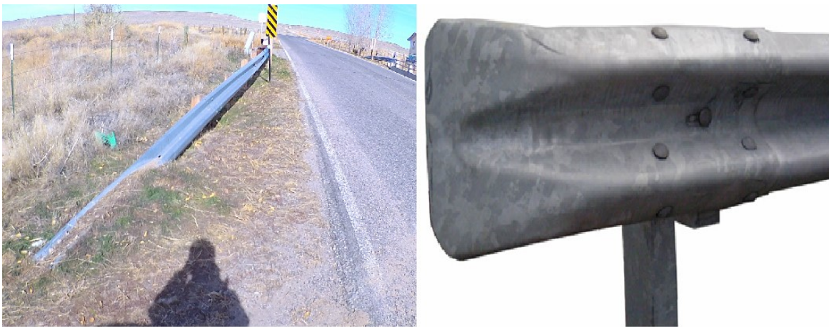
Figure 2. Typical turned-down (left side) and blunt-end (right side) terminals which became popular in the early 1960s.
