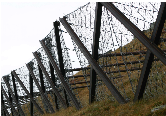
Fig. 3. Semi-rigid snow supporting structure at Val Thorens Ski Resort, France.
