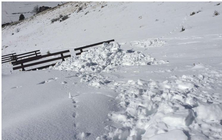
Fig. 5. Avalanche debris resting on SSS at the Milepost 151 Avalanche site.
