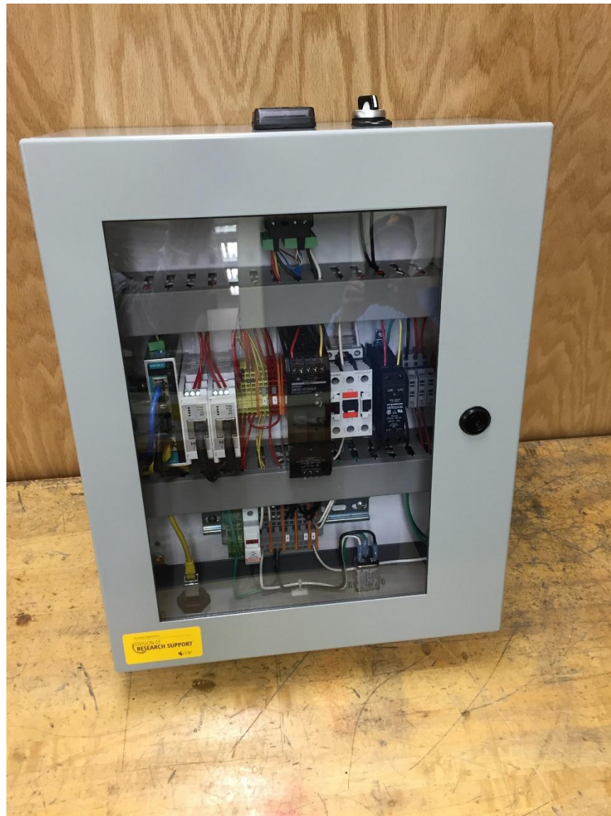
Figure 8: A typical modern data acquisition unit.
